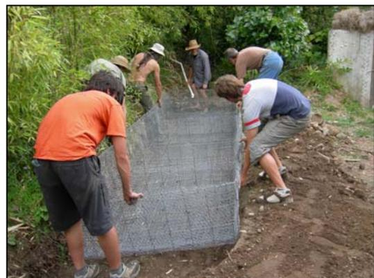
The frame is built using baffles, so that the water is forced to take the longest route possible, snaking over one section of the tank and under the next. The concrete wire is used for its
